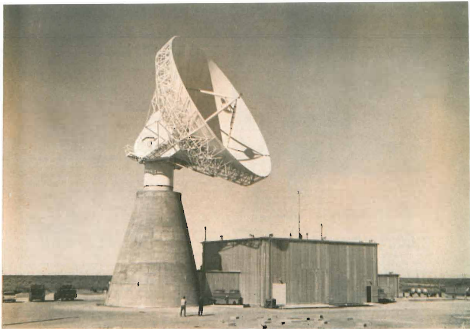
Typical of the radars used for signature analysis is this advanced projects terminal measurements radar built by Raytheon for the White Sands Missile Range in New Mexico.
